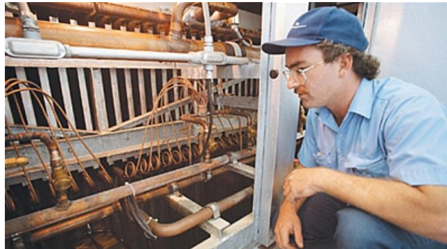
Figure 2. Custodian inspects heating unit.
