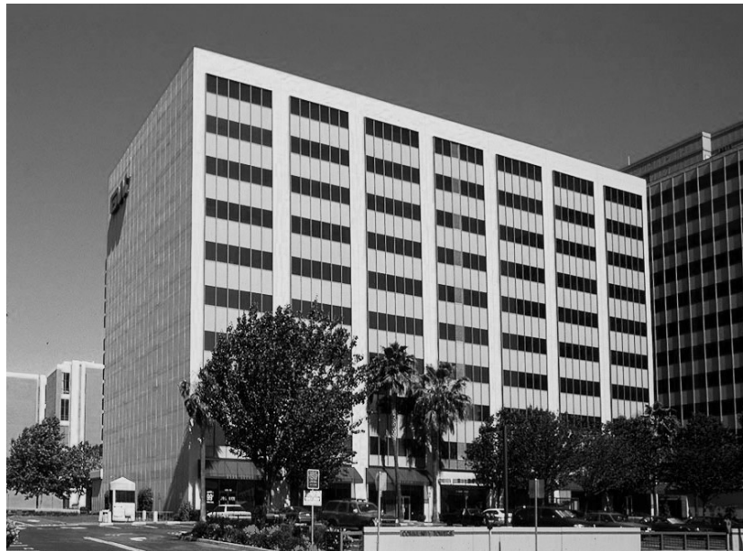
Figure 1. Community Towers Complex.
