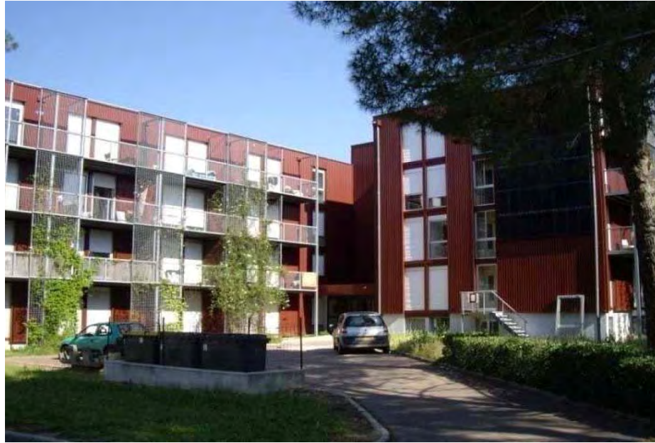
Figure 1. South view of the building after retrofitting.
