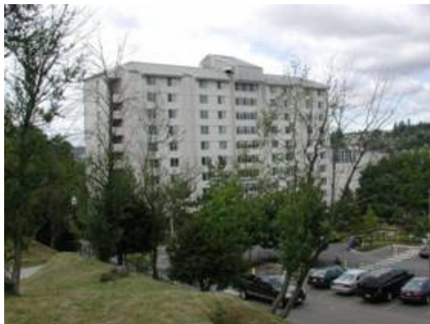
Building 865 NB Kitsap Bremerton, WA
